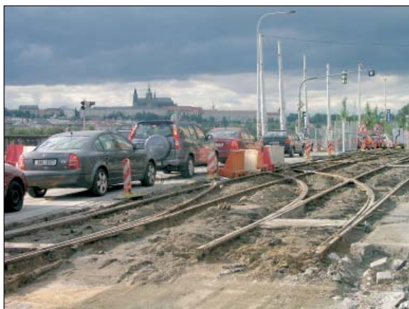
Repair starts on the Palackého square crossroads and superstructure panels are replaced on the tramway line in the Lidická street
