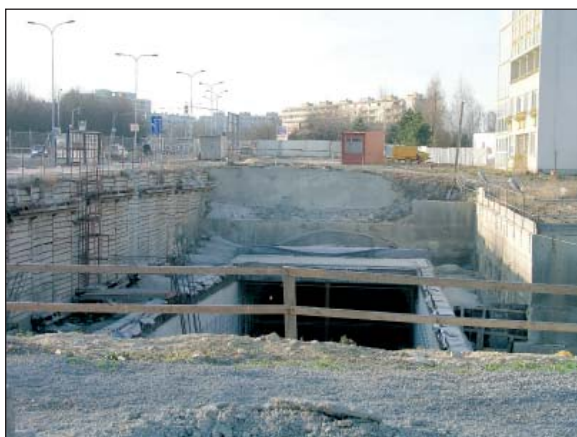
An open ditch for Metro at the Liberecká bus stop
