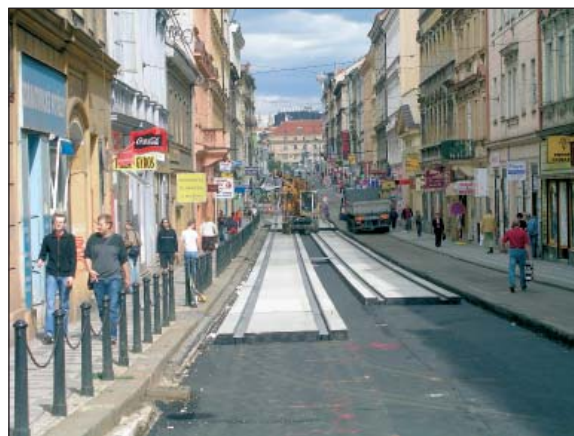
Repair starts on the Palackého square crossroads and superstructure panels are replaced on the tramway line in the Lidická street
