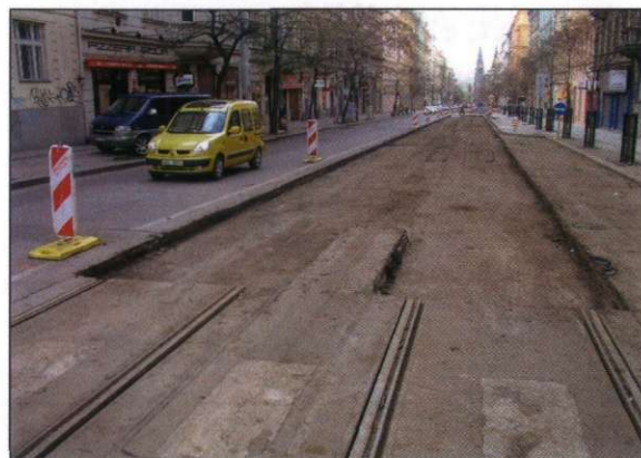
A tram line redevelopment on the Olšanská and Korunní streets
