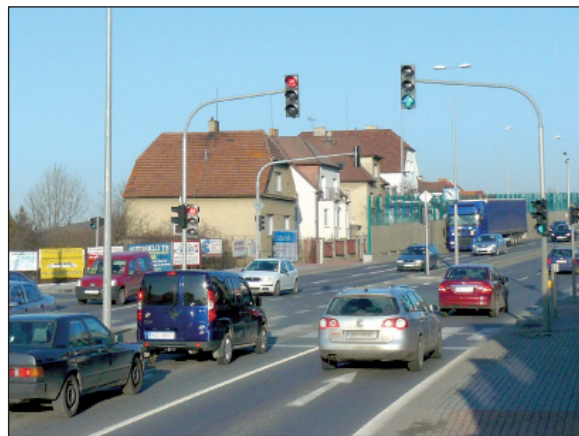
Intersection Karlovarská – Drnovská renovated from source OPD
