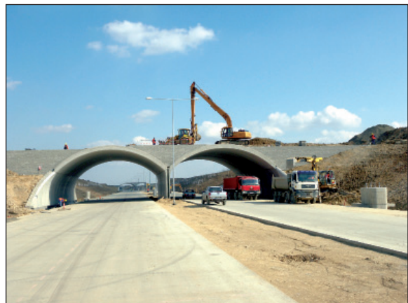
Prague Outer Ring Road – construction near Cholupice
