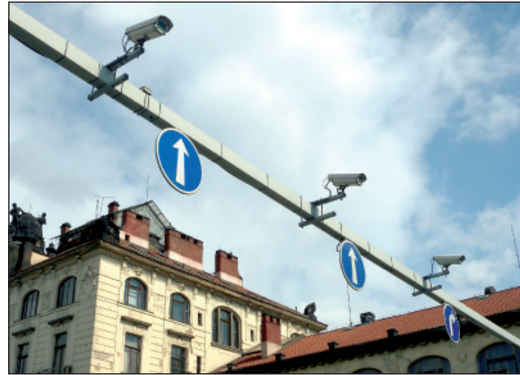
Spot strategic detectors on Francouzská Street and sectional strategic detectors on Wilsonova Street
