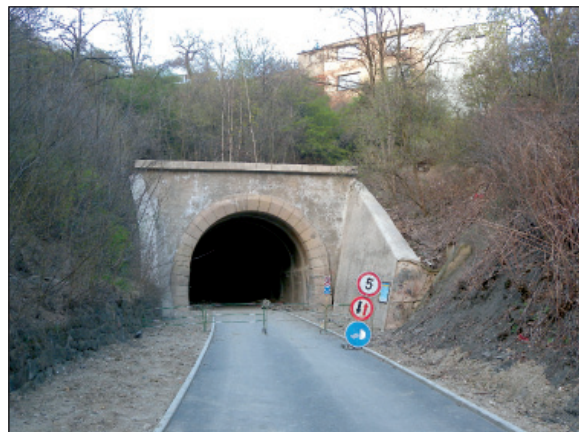
Seifertova – Vítkov Tunnel – Balabenka cycle track under construction
