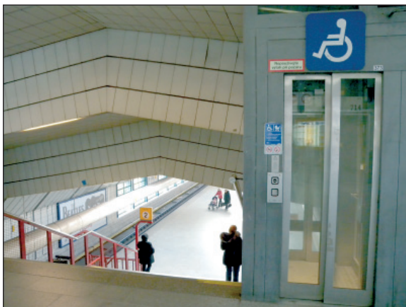
Passenger elevator at Luka station on "B" Line
