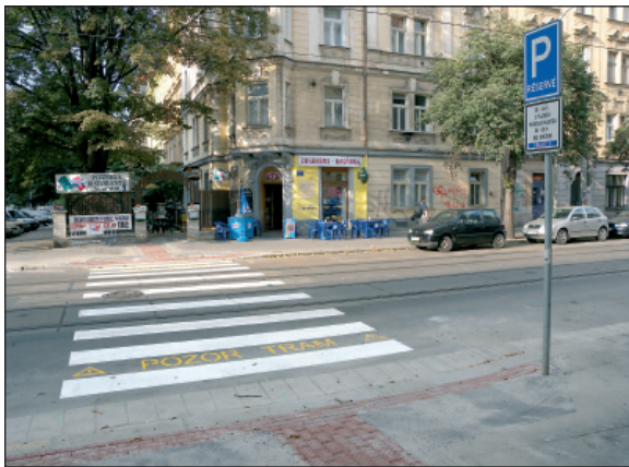
Renewed crossing with added warning
