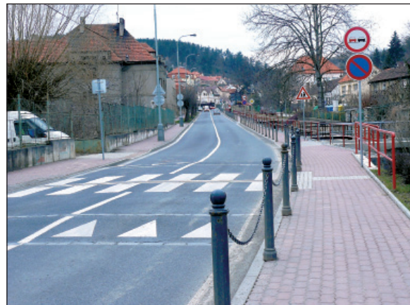
Starochuchelská after carriageway and pavement renovations
