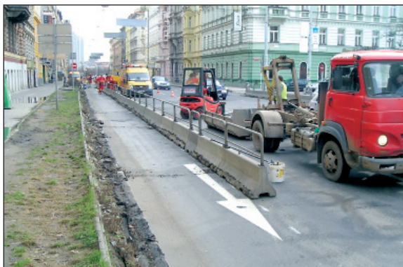
Legerova Street – assembly of concrete barriers
