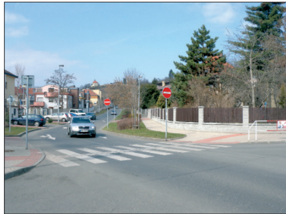
New pavements on Trojská Street
