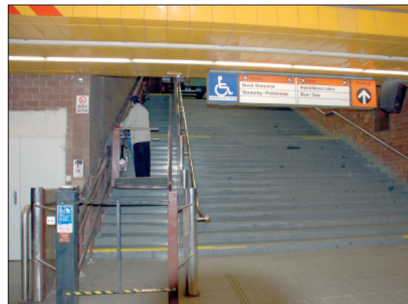
Stair lift at Nové Butovice station on "B" Line
