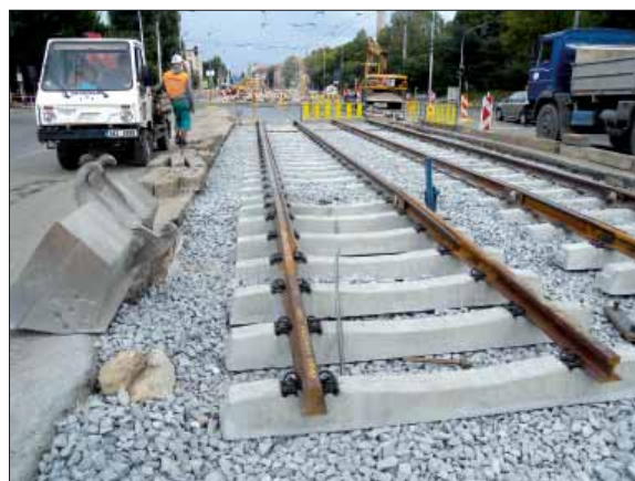
Changeover from grooved to new flat bottom rail by Kotlářka stop
