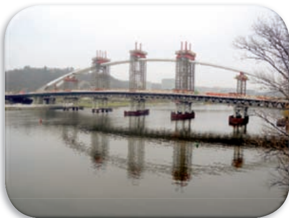
Construction of Trojský most
