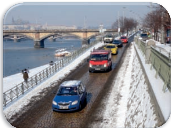
Temporary embankment road during repairs on Rašínovo nábrží.
