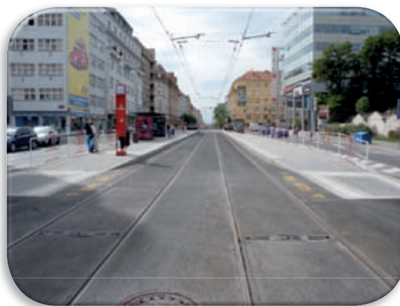
Flora tram stop after refurbishment
