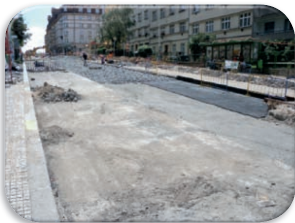
Summer repairs on Jičínská street
