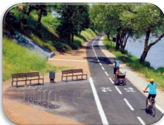
Malá Chuchle – Barrandovský most cycle track
