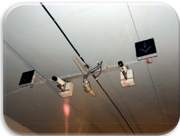
Cameras and LED signals in Blanka
