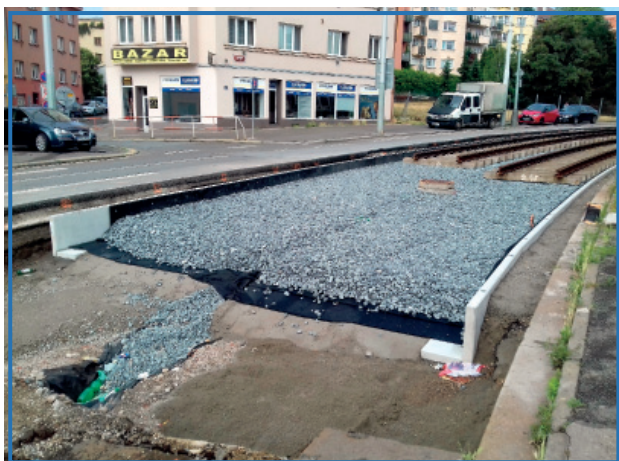
Track refurbishing at the intersection Zenklova – Primátorská
