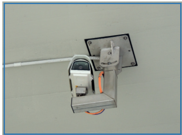
Television surveillance camera in the tunnel
